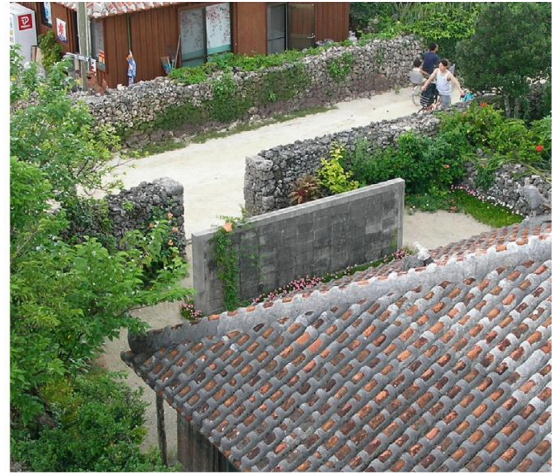
Image 1 (left): Streetscape of the Ryukyu islands; a typhoon barrier of coral stone walls and trees (Okubo, 2016). Image 2 (right): Visible are the coral stone walls, the Hinpun and the red roof tiles bonded with plaster (Okubo, 2016).
