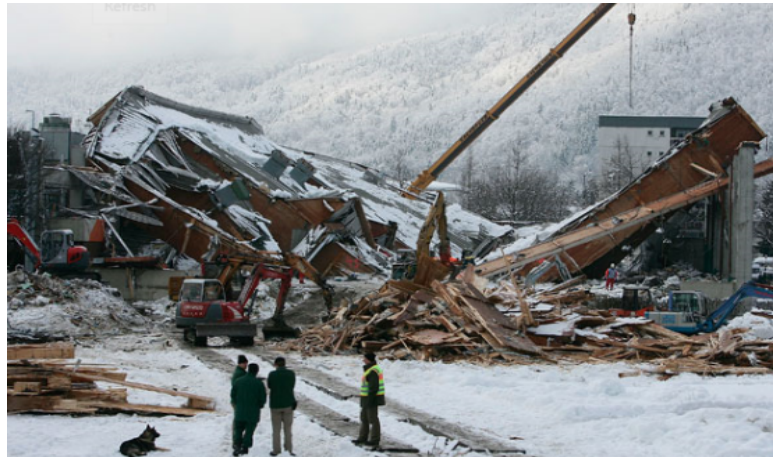
Figure 4.6: Collapse of the ice skating arena in Bad Reichenhall. Credit: www.calgaryherald.com
