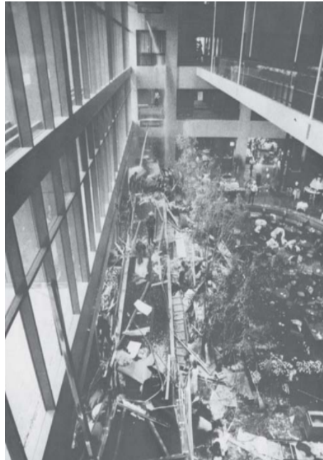
Figure 4.4: Hyatt regency walkways collapse [46]
