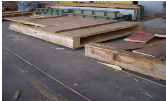
Figure 4.7: Box girder components of the ice skating roof [82]
