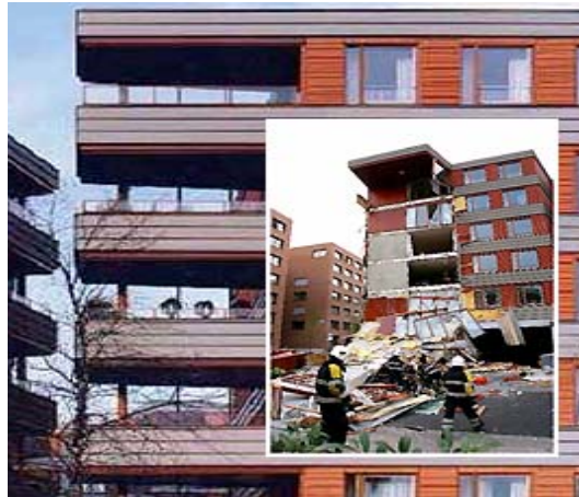
Figure 4.12: Collapse of the balconies of the Patio Sevilla apartment. Credit: www.architectenwerk.nl
