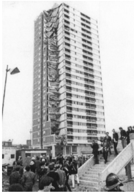
Figure 4.20: The collapse of Ronan Point apartment [11]
