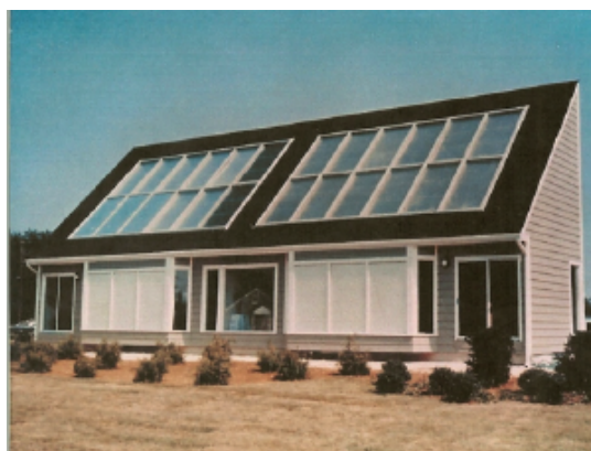
Figure 1.1: An image of Solar One, a house that used solar energy for its heating and electrical requirements. It was built with support from Delmarva Power and Light by the Institute of Energy Conversion in 1973 [1].
