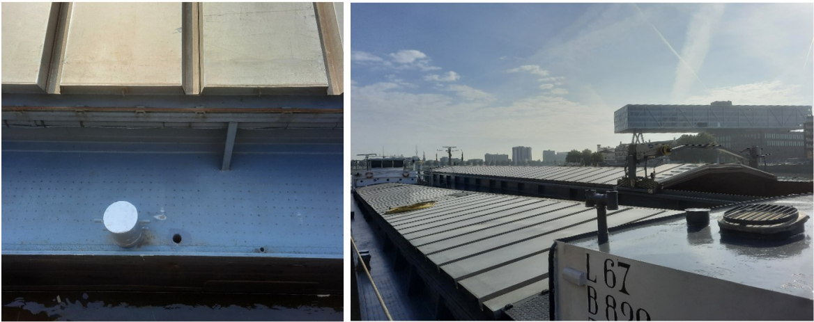
Figure 3.26: Field survey towards mounting spacing
