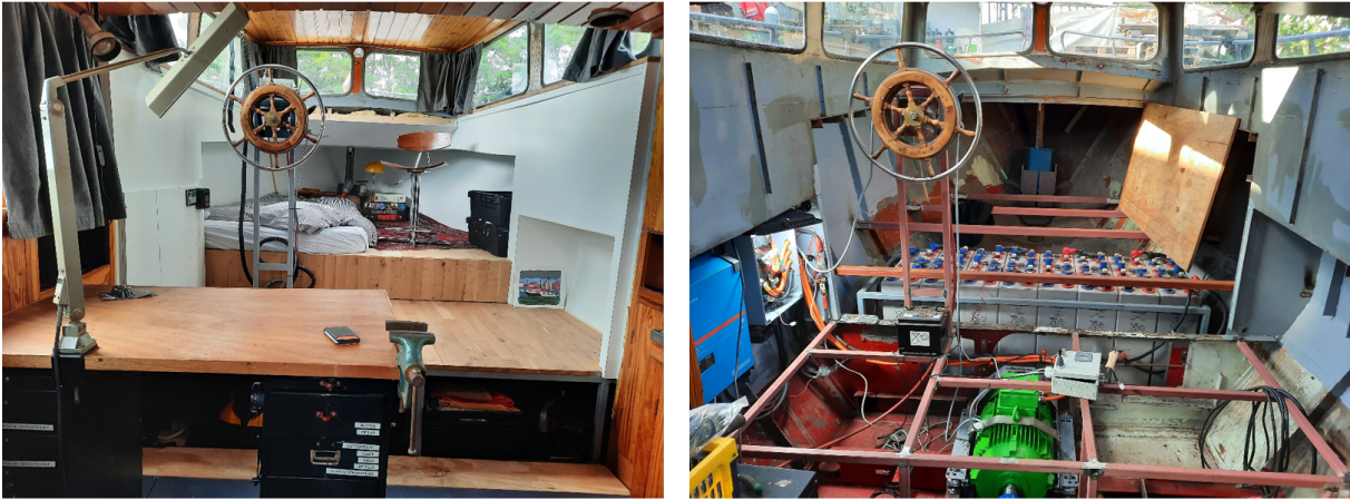
Figure 3.29: Harmonie electrical engine and batteries
