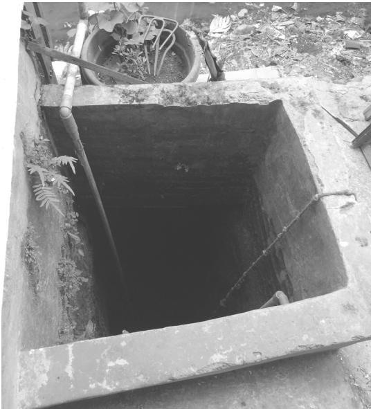
Img 06.25 (right) - New connection to the water supply (Source: Authors own)
