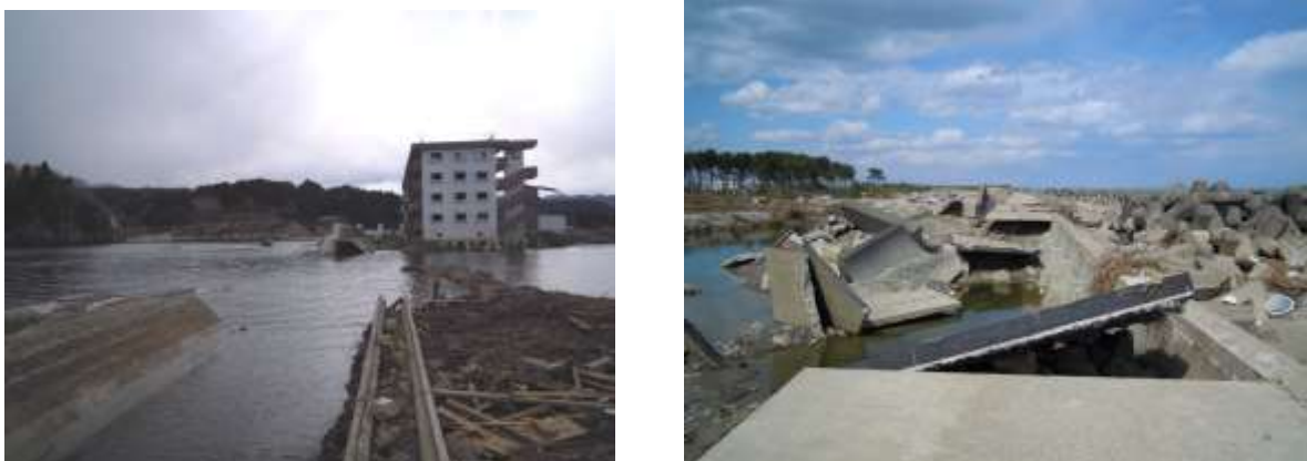
Fig. 1. Failure of coastal dykes along the Tohoku coastline. In many places the dykes were completely breached (left), or suffered heavy scour (right).
