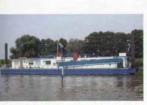
The water quality is measured 24 hours a day at different stations along the rivers Rhine and Meuse. The picture presents the monitoring-station at Lobith.
