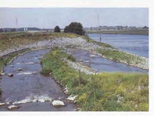
Fish passage along the river Meuse near Roermond. Through such fish passages, fishes can pass along a weir or sluice.
