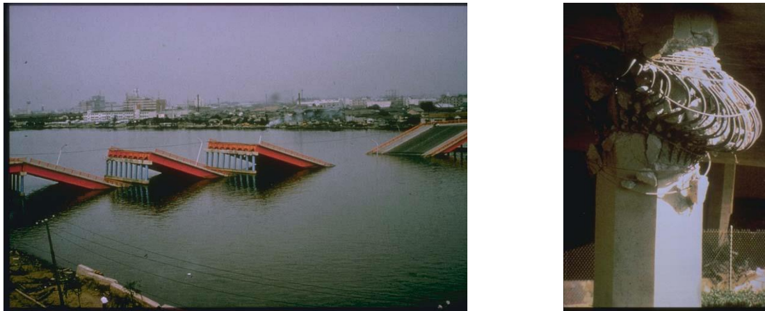
Figure 2. Unseating of bridge deck (left). Shear failure due to insufficient detailing (Courtesy of NOAA/NGDC)
