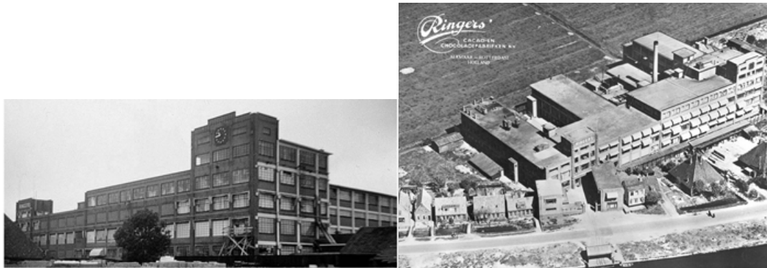
Figure 4. Façade 1937 and Aerial view 1940
