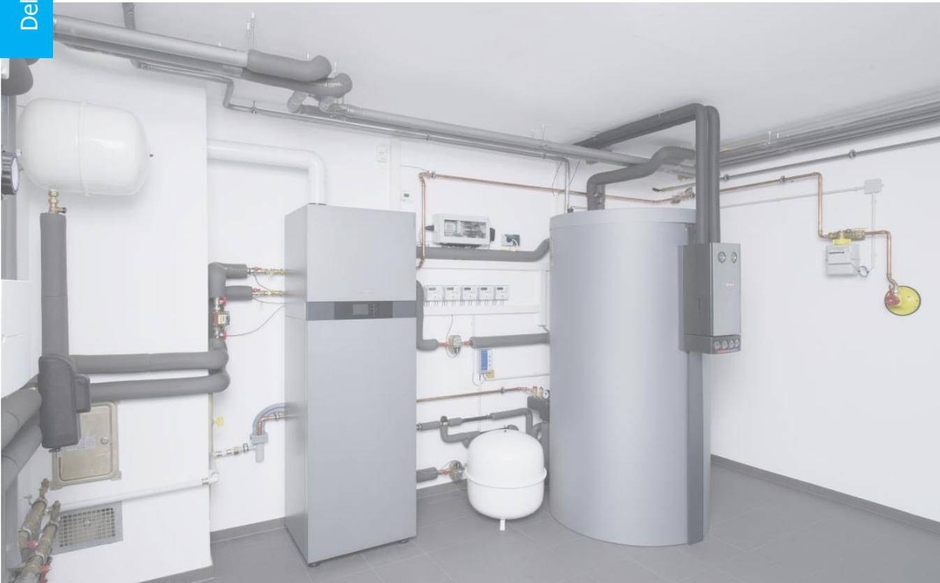
Photo: Boiler heated by adsorption driven heat pump using zeolites, in tandem with a gas heater and environmental heat (produced by Viessmann Werke GmbH & Co KG)
