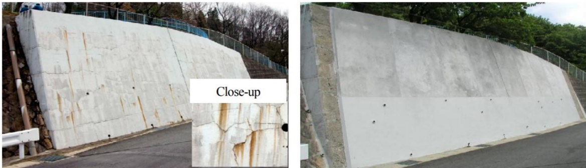
Figure 6. Surface repair with SHCC of a concrete retaining wall in Gifu [37].
