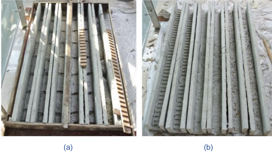
Figure 16. Fabrication of SHCC U-shaped permanent formwork; before casting the bottom plate (a) and after demoulding (b) [88].
