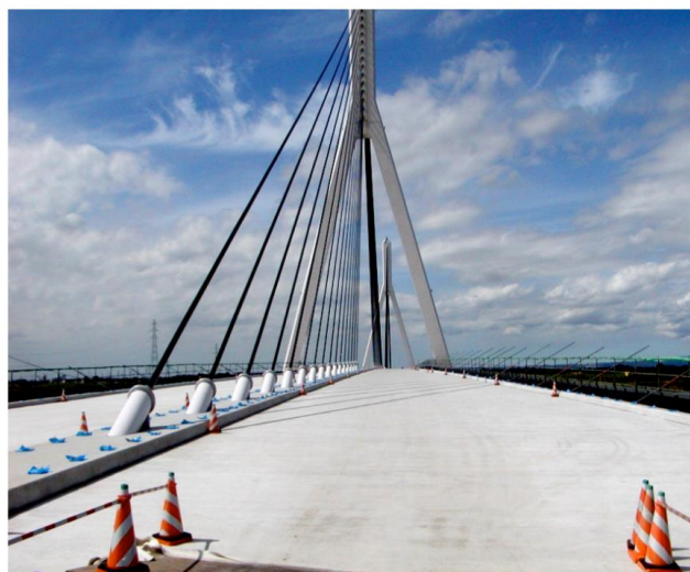
Figure 5. Mihara bridge with SHCC/steel composite deck (Hokkaido, Japan, 2004).
