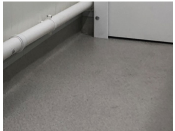
Figure 133: Linoleum floor with plinth
