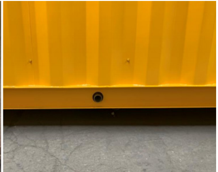
Figure 136: Central outlet drains
