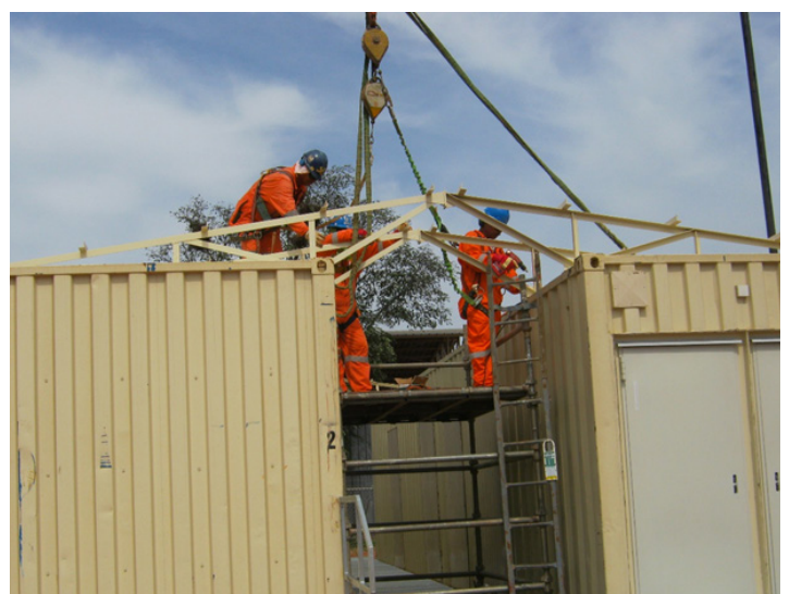
Figure 120: Container construction by Kan Bud
