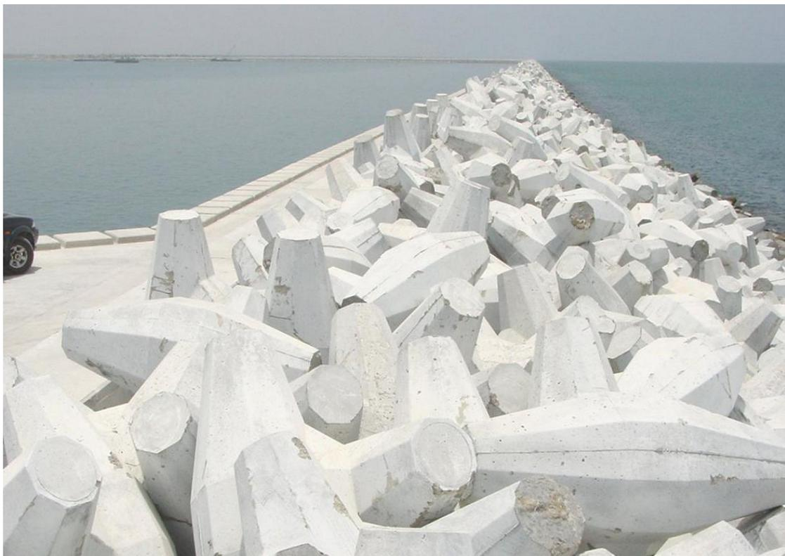
Figure 3 Breakwater armoured with Core-loc® elements
