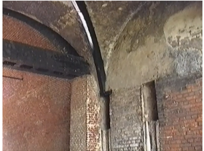
Fig.4 A Screenshot of a Video Taken in 1995, Showing the Degradation of Building Due to Excessive Water.
