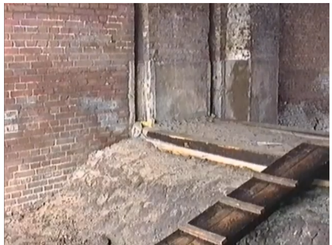
Fig.5 A Screenshot of a Video Taken in 1995, Showing the Degradation of Building Due to Excessive Water.
