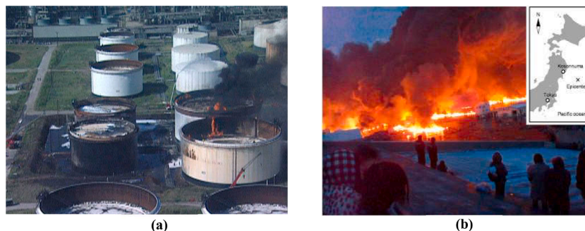
Fig. 1. Post-earthquake fires related to chemical process industry. (a) Massive fires at the TUPRAS Izmit refinery in the 1999 Kocaeli earthquake [6] (b) Oil spill fires at Kesennuma Bay in the 2011 Great East Japan Earthquake and Tsunami [8].
