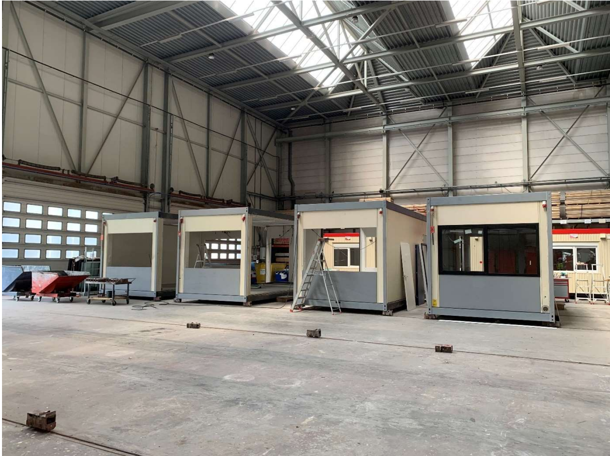
Figure 8 Refurbishment of used temporary office units at Daiwa (own picture)
