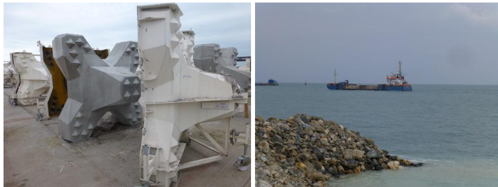
Figure 6-14. Breakwater extension, Port of Constanta, Romania, 2013
