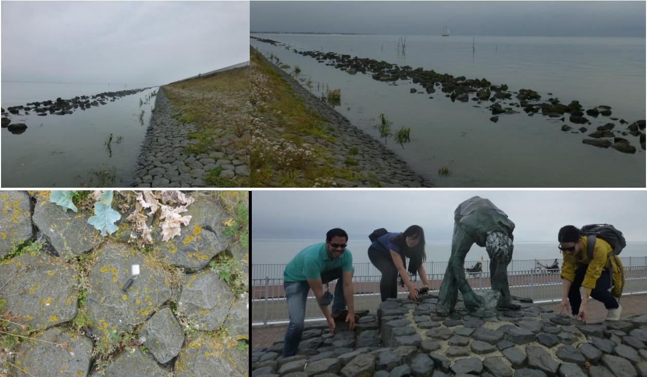
Figure C- 6. Afsluitdijk outer slope and basalt columns details
