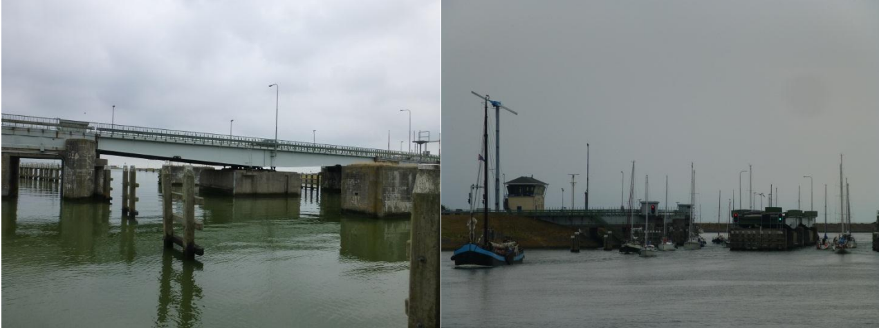
Figure C- 8. Kornwerderzand swing bridge on the A7 highway
