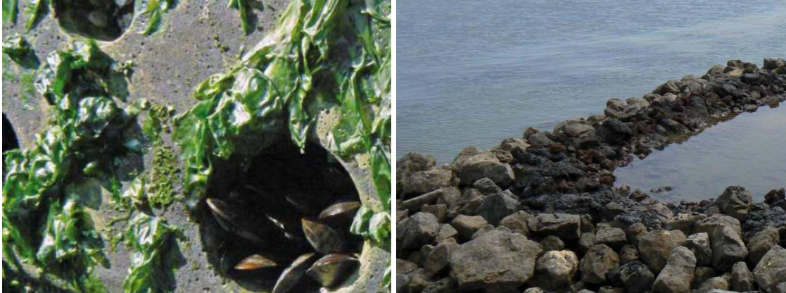
Figure 7-29. Eco-Concrete in Ijmuiden (left) and tidal pools in the Eastern Scheldt dike (right)
