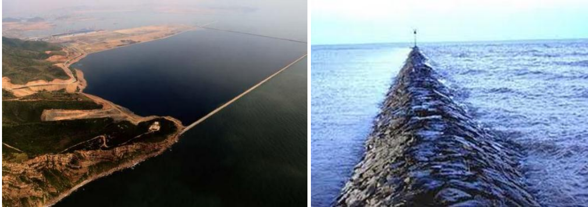
Figure 6-10. South Breakwater , Hulushan Bay, Dalian City, China, 2012
