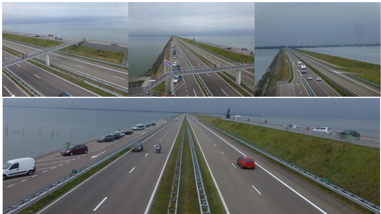
Figure C- 5. Pedestrian bridge and views of the dike to Noord Holland direction
