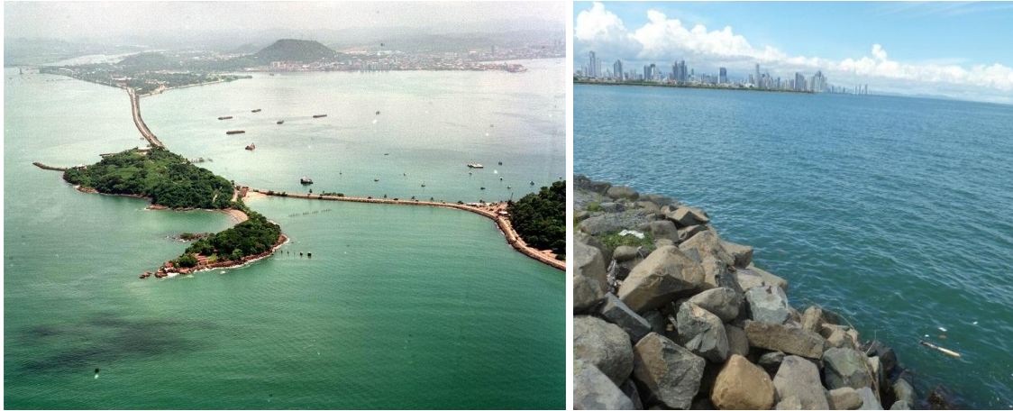
Figure 6-1. Amador Causeway rubble mound breakwater, Panama city, Panama, 1913
