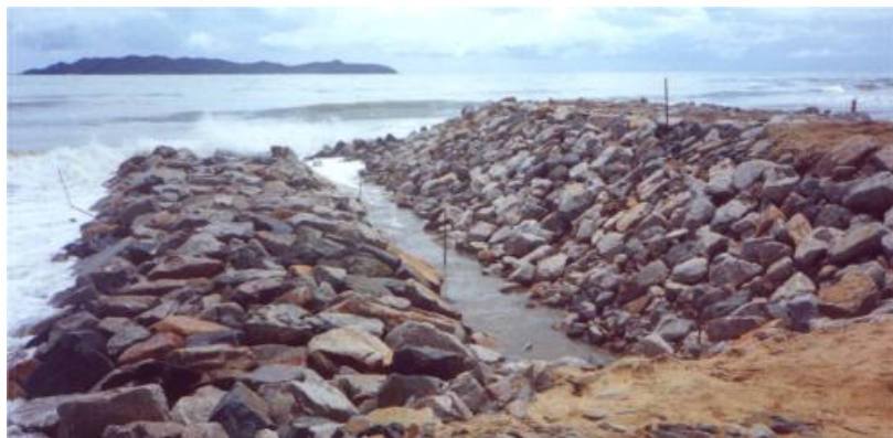
Figure 6-9. Berm breakwater
