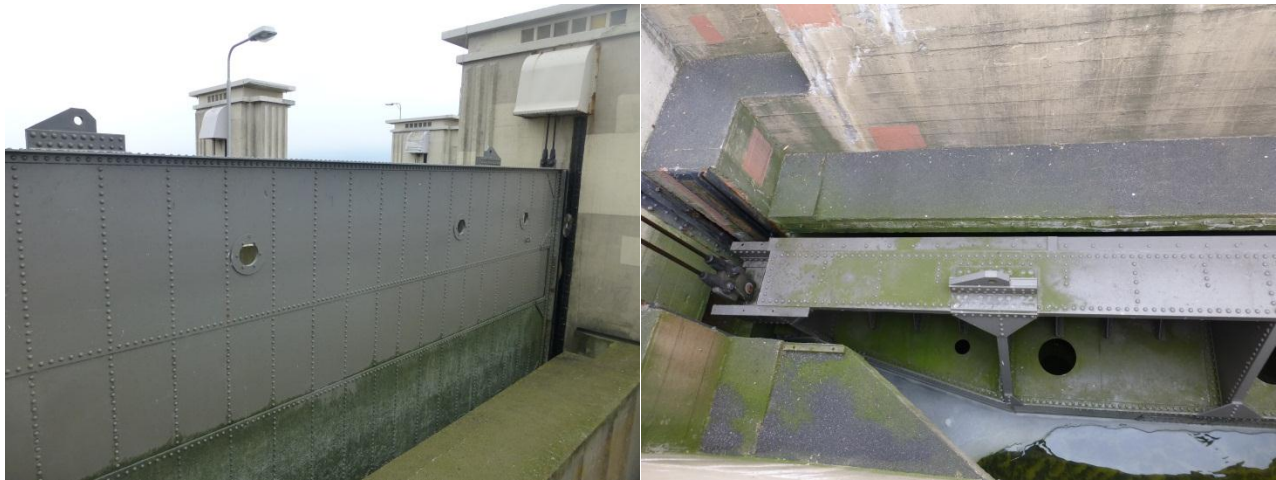
Figure C- 11. Lorentz Sluizen complex - Lifting gates
