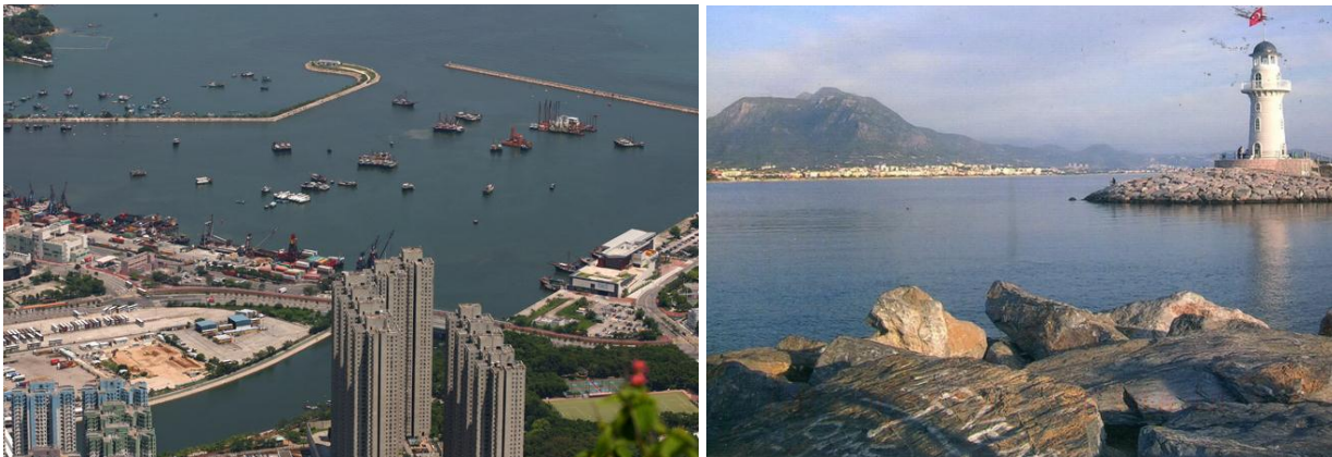
Figure 6-11. South Breakwater of the Typhoon Shelter at Hei Ling Chau, Hong Kong, China, 1993
