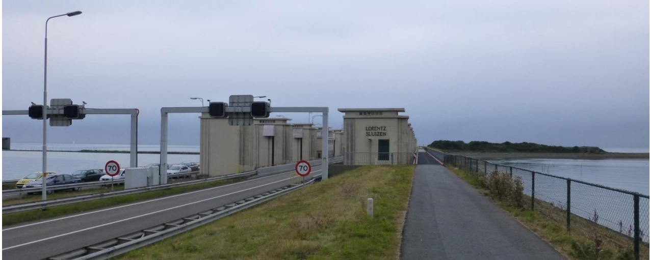
Figure C- 10. Lorentz Sluizen complex - Double set of lifting gates
