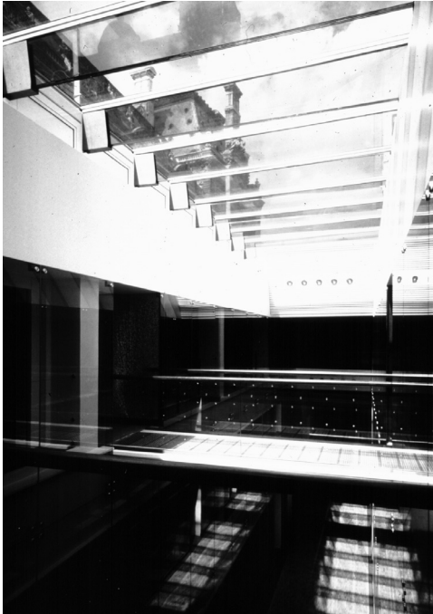
Fig. 5.2 Laboratoires des Grand Louvre, Paris. Span 4.6 m, 4 layers (4x15 mm), PVB laminated, annealed. 1991. Structural glass engineer: RFR, Paris, France.
