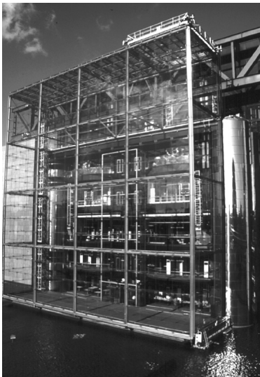
Fig. 1.24 Serres of the National Museum of Science, Technology and Industry in the Parc de la Villette, architectural design by Adrien Fainsilber, structural glass design by RFR, 1986, Paris, France.
