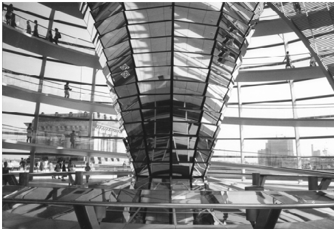
Fig. 1.6 Reichstag renovation and extension, architectural design by Norman Foster & partners, 1999, Berlin, Germany. Interior view of the glass covered dome, on the left part of the Reichstag building, on the right a view over Berlin city. The mirror clad pillar in the centre reflects daylight into the main meeting room of the German parliament.
