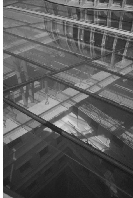
Fig. 5.3 Roof of the renovated ING Office, Budapest. Span 4.5 m, 3 layers (8-12-8 mm), PVB laminated, annealed & thermally tempered. 1994. Structural glass engineer: ABT, Velp, the Netherlands.
