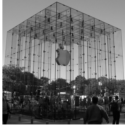
Fig. 1.27 Glass cube over the entrance to the Apple Store on 5 th Avenue, architectural design by Bohlin Cywinski Jackson, glass design by Eckersley O'Callaghan, 2006, New York, USA.
