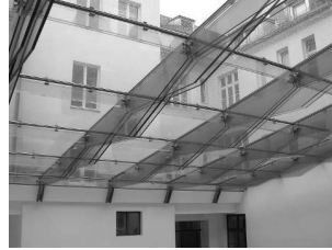
Fig. 5.7 Atrium roof of the Chamber of Commerce, Munich, Germany. Total span 14 m, 5 segments (2 double, 3 triple), double and triple layers, PVB laminated, thermally tempered and heat strengthened, 2002. Structural glass engineer: Ludwig und Weiler, Germany.
