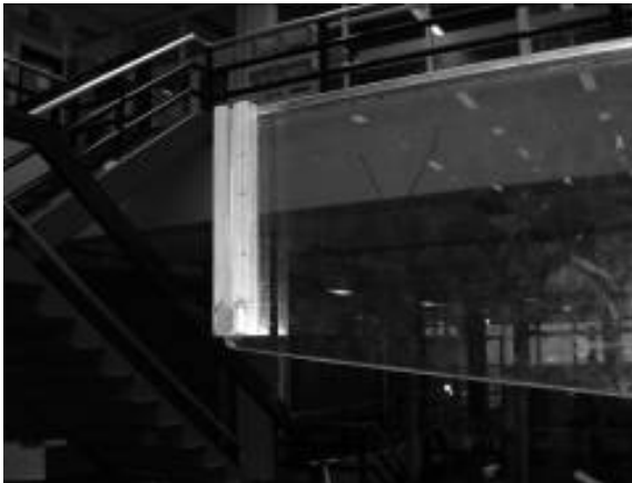
Fig. A.14a, b Aluminium transitional components glued to the main beam (a, left) and to the purlins (b, right).
