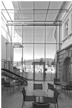
Fig. 5.14a Glass roof at the Spa Thermen in Badenweiler. Span: 6.2m. 3x10 mm thermally toughened glass. PVB laminated. Steel reinforced and post-tensioned. 2004. Structural glass engineer: Schlaich Bergemann, Stuttgart, Germany.
