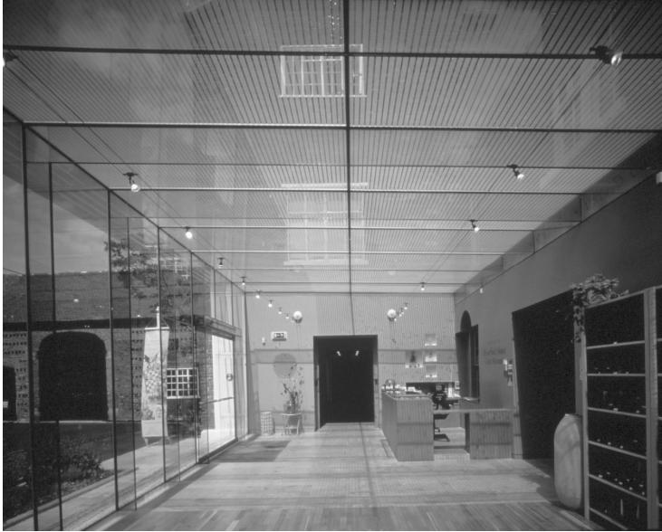
Fig. 5.1 Broadfield House Glass Museum extension, Dudley West. Span 5.7 m, 3 layers (3x10 mm), resin laminated, thermally tempered. 1994. Structural glass engineer: Dewhurst Macfarlane, London, UK.
