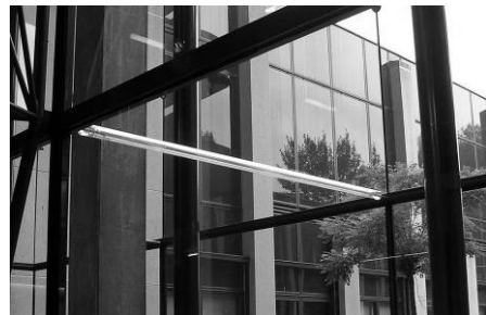
Fig. 2.2 Transparent Façade Strut in an extension of the TU Delft Architecture Faculty (impression).
