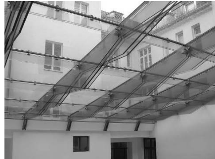
Fig. 8.7: Atrium roof of the Chamber of Commerce, Munich, Germany. Total span 14 m, 5 segments (2 double, 3 triple), double and triple layers, PVB laminated, thermally tempered and heat strengthened, 2002. Structural glass engineer: Ludwиг und Weiler, Germany.
