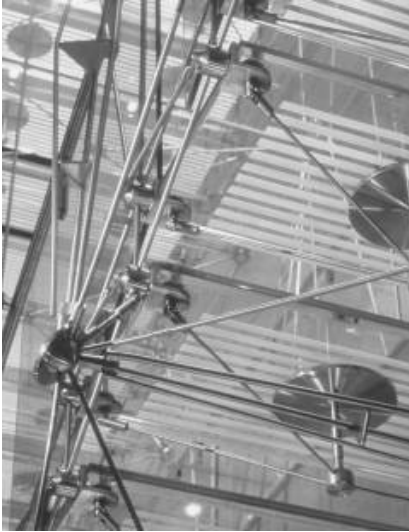
Fig. 1.16 Joseph store staircase, architectural design by Eva Jiricna, glass design by Tim Macfarlane, 1989, London, UK.
