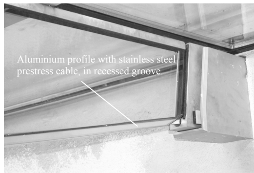
Fig. 8.18 Glass beam (detail) at the Spa Thermen in Badenweiler.
