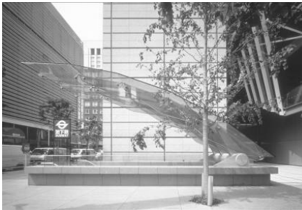
Fig. 1.18 Yurakucho canopy, architectural design by Rafael Viñoly, glass design by Tim Macfarlane, 1997, Tokio, Japan.
