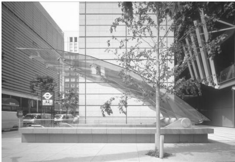
Fig. 8.6: Subway Entrance Canopy, Tokio, Japan. Total span 10.8 m, 4 segments (3 of which double), two 19 mm thermally tempered glass layers, with an acrylic layer in between, 1996. Structural glass engineer: Dewhurst Macfarlane, London, UK.
