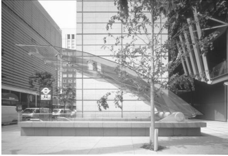
Fig. 5.6 Subway Entrance Canopy, Tokio, Japan. Total span 10.8 m, 4 segments (3 of which double), two 19 mm thermally tempered glass layers, with an acrylic layer in between, 1996. Structural glass engineer: Dewhurst Macfarlane, London, UK.
