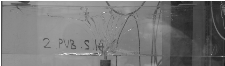
Fig. 9.7a Only in fully predamaged double layer PVB laminated heat strengthened glass beams some post-initial failure resistance remains.
