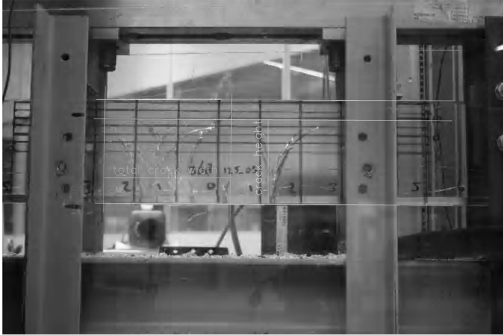
Fig. I.5 Photograph of initial crack pattern of specimen GB368-03 in Autocad. Determination of crack related results crack height and total crack width (upon initial failure).
