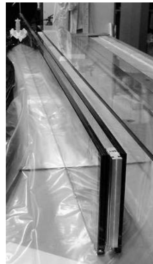
Fig. A.14a, b Aluminium transitional components glued to the main beam (a, left) and to the purlins (b, right).
