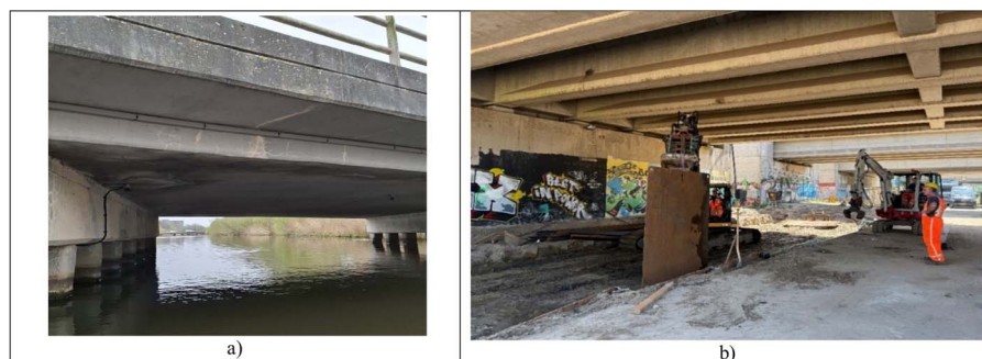
Figure 3 Photos of (a) a reinforced concrete slab bridge and (b) a prestressed concrete girder bridge
