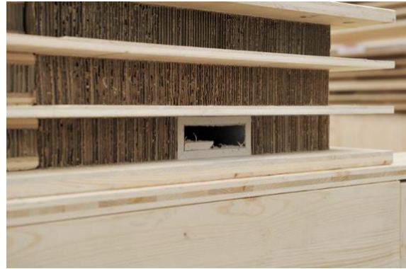
Figure 5.17. A cable canal for wiring integrated in a three-layered ceiling panel (ECOCELL, n.d.).
