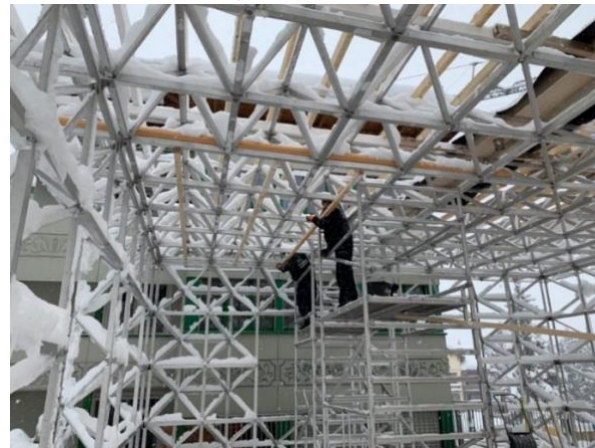
Figure 5.11. On site assembly of the Wonderframe structure (C2C Centre, 2019).
