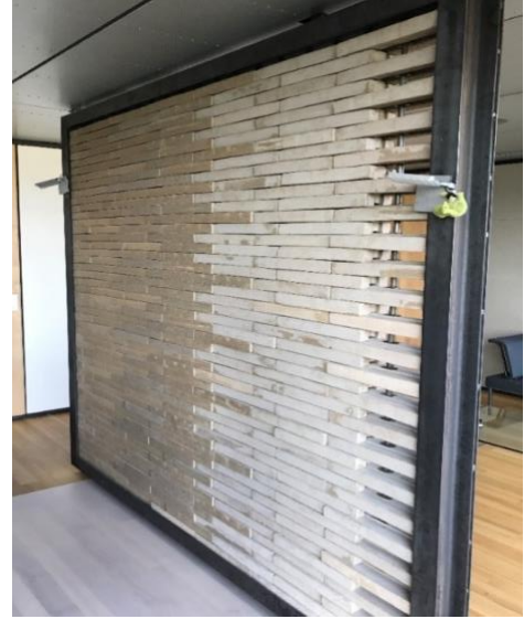
Figure 5.6. A dry-stacked turning wall created using wasted based bricks (own photo).
