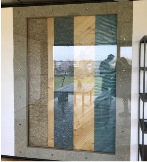
Figure 5.5. Wall intersection showing different layers of insulation (own photo).
