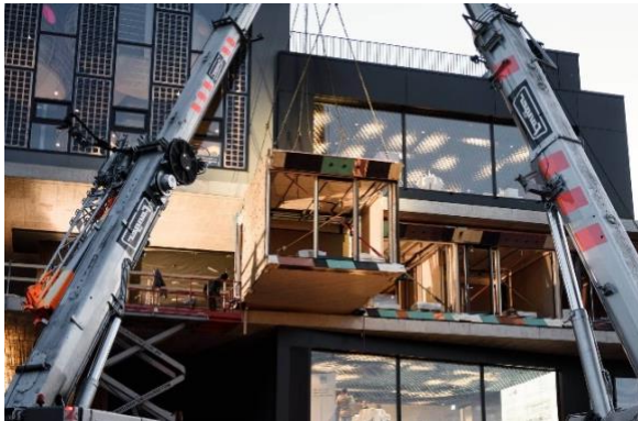
Figure 5.3. On-site assembly of the modules with two mobile cranes (Kaufmann, 2017).
