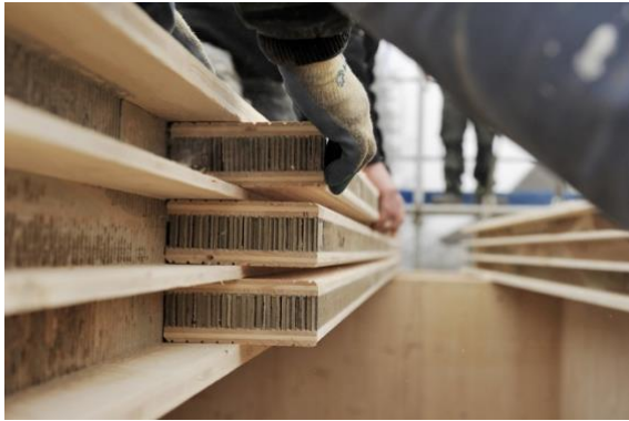
Figure 5.16. A ceiling consisting of a three-layered panel with tongue-and-groove connection (ECOCELL, n.d.).
