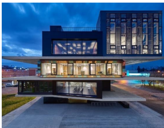
Figure 5.1. The UMAR unit located on the second floor of the NEST building © Zooley Braun, Stuttgart (Sobek et al., 2018).
