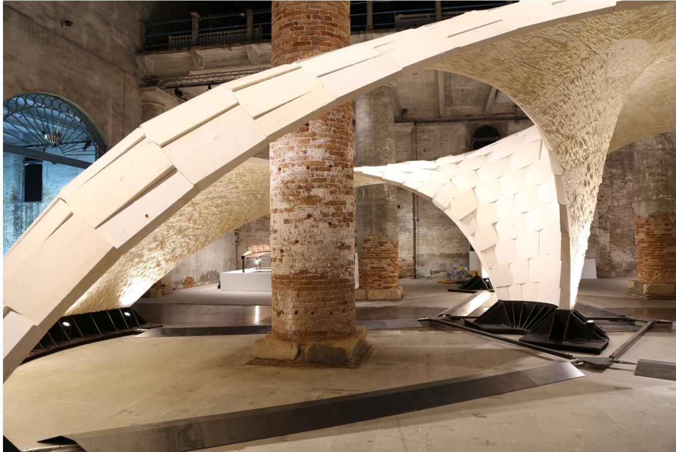
The Armadillo Vault, showing a fixed support and tension-based foundation creating a compression ring effect. (Frearson, 2017)
