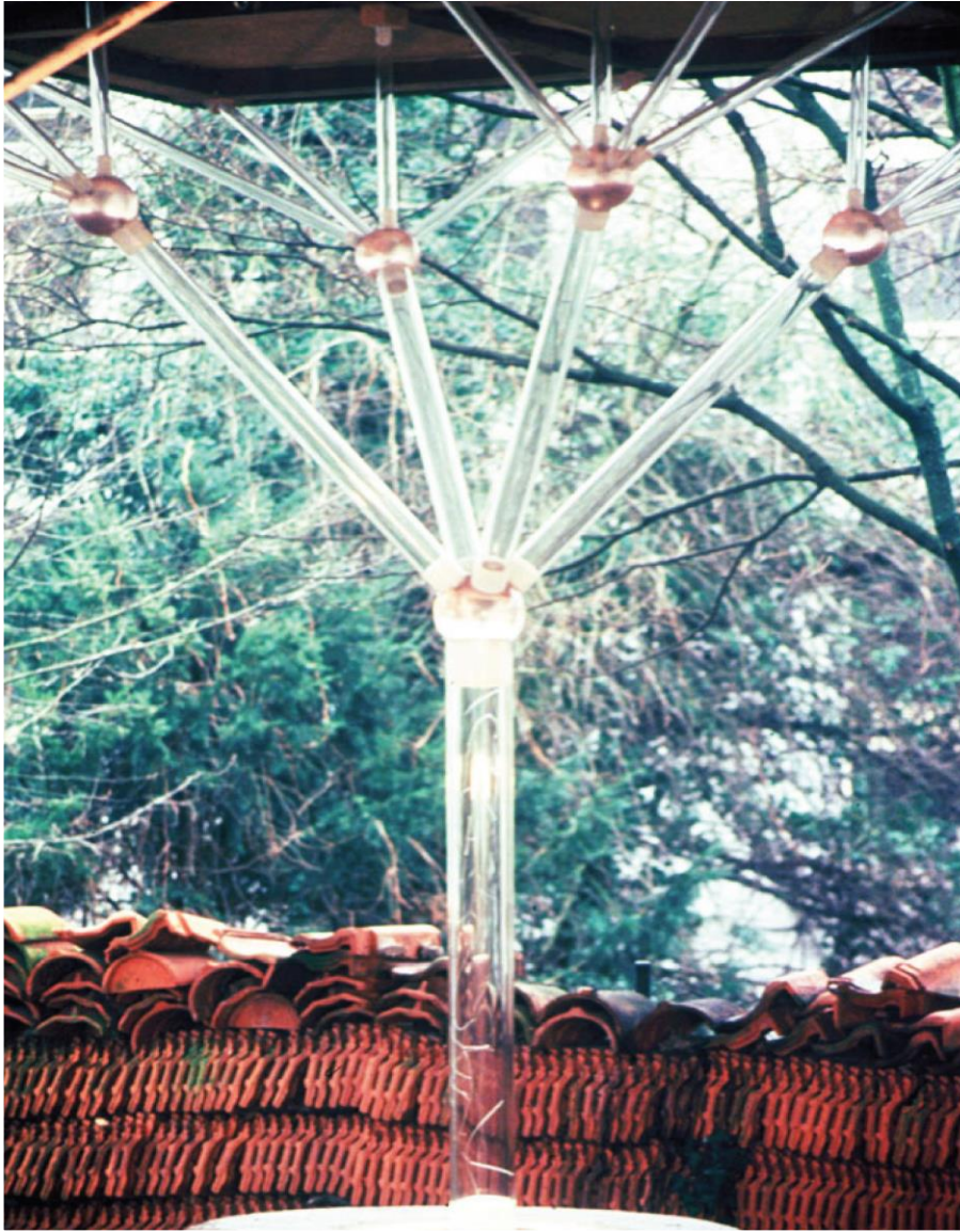
Tubular extruded glass column tree structure in Aachen, Germany for (Knaack, 1998)
