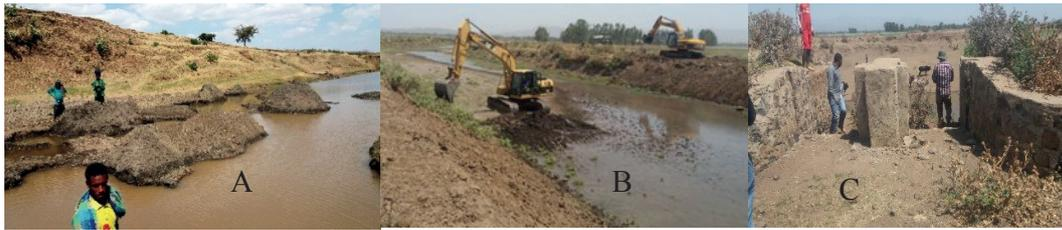
Figure 2.15. (A) Excavated sand accumulation by sand miners in the Middle River Reach. (B) River channel enlargement and deepening to increase flow conveyance. Excavated material is used further downstream for embankment construction. (C) Flood outlet structure to the farmlands as low height weir (April, 2016).
