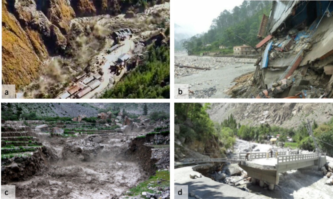
Figure 1: Destructive downstream impact of GLOFs. (a) India 2021 (retrieved from https://theshillongtimes.com ) , (b) India 2012 (retrieved from https://climatechangenews.com ), (c) Nepal 2011 (Photo from Astrid Hovden), (d) Pakistan 2019 (retrieved from https://dawn.com )
