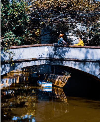
Figure 1-29 Historical bridge in Lijiao, Guangzhou. Captured by the author
