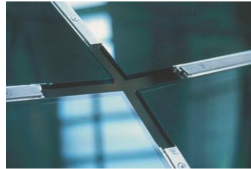
Figure 58 Linear connections in both the meridian and ring directions, positioned at the panel corners (Wurm, 2007)
