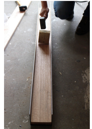
Figure 198: Hammering the hardwood board into the U-profile (own work, 2025).
