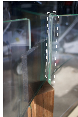
Figure 208: Application of clear silicone tape along the slot edge to prevent glass-to-glass contact (own work, 2025)
