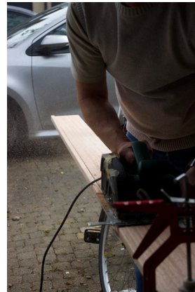
Figure 197: Cutting the hardwood board to size (own work, 2025).
