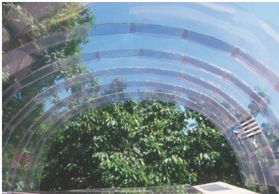
Figure 54: Segmented three-pinned arch structure (Wurm, 2007).
