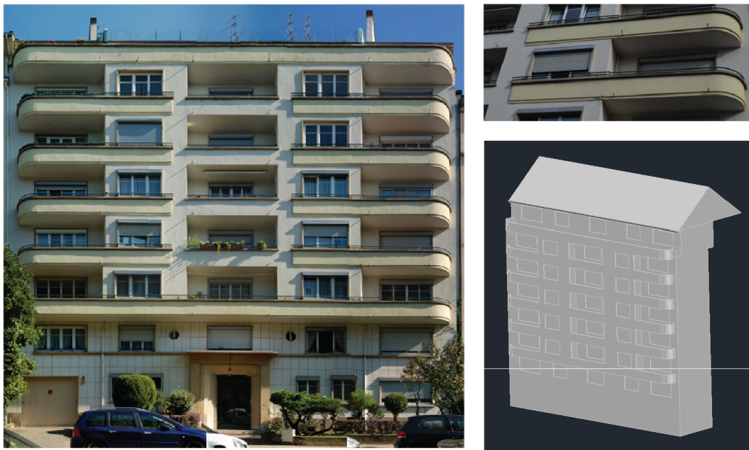
FIGURE 3.3: Rue de l'Argonne 4 facade features and model show the extreme shape of the balconies and complex result in the 3D model
