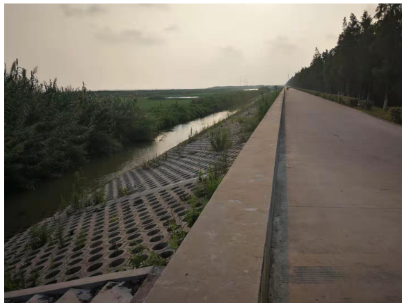
(c) Third type of outer slope structure
