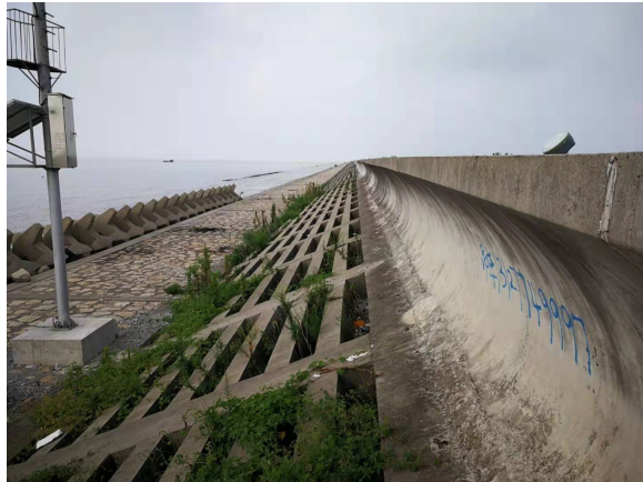
(a) Sea wall structure at Location A
