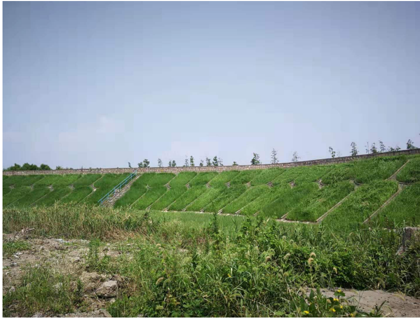
Fig. A.16.: Grass cover on the inner slope
