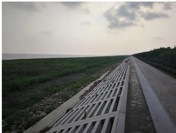
(b) Second type of outer slope structure
