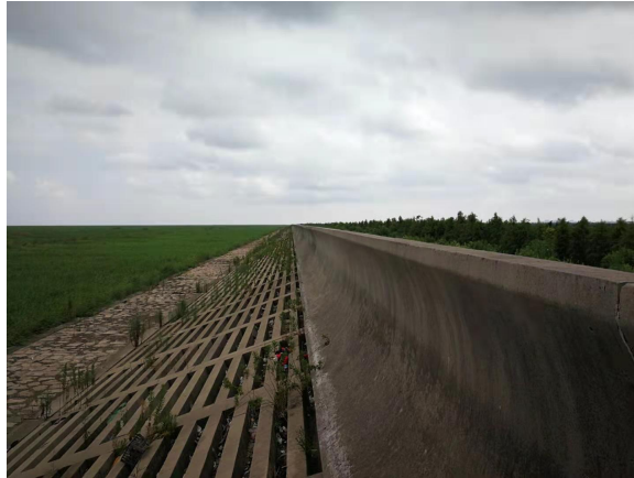
(a) Typical sea wall structure
