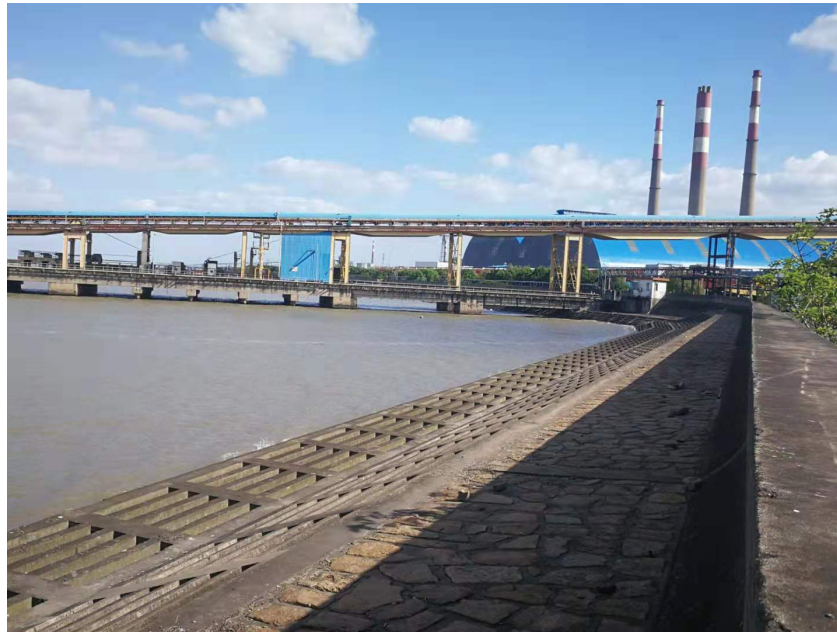
Fig. A.2.: Sea embankment near Sujian Wharft
