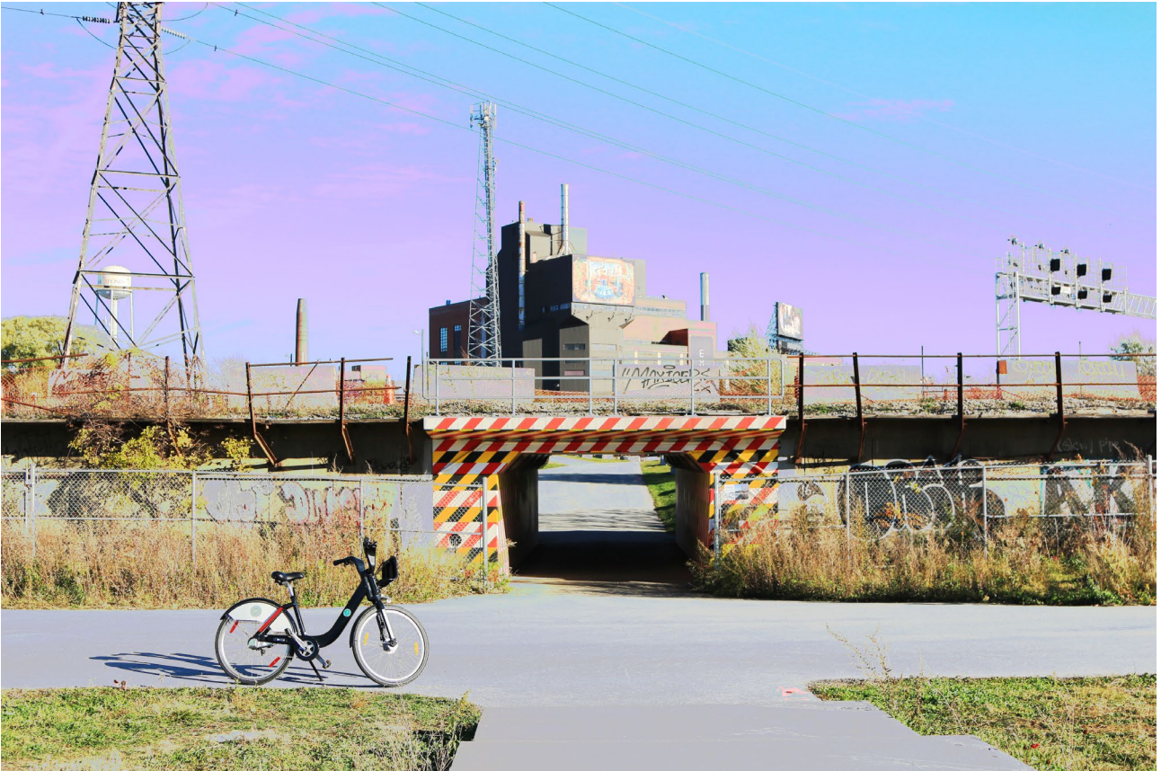
Lower Don Tunnel Entrance Source: by Author
