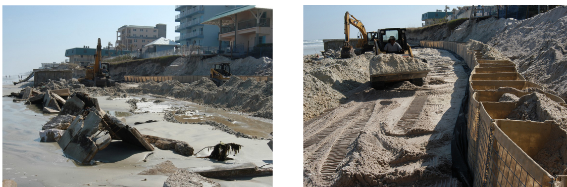
Figure 1.1: Beach erosion and property damage due to Hurricane Jeanne (2004) at New Smyrna Beach (left). The filling of sandbags which act as a temporary seawall (right).
