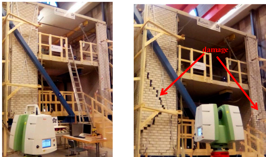
Figure 4. On the left: the masonry wall before the seismic testing; on the right: the damaged masonry wall after the seismic testing.
