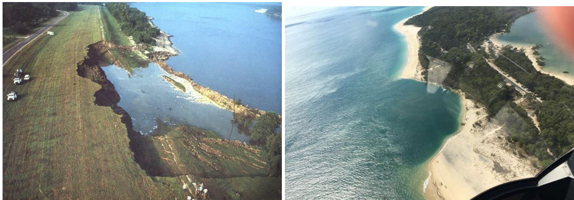
Figure 1. Damage to a river dike caused by a flow slide, from US Army Corps of Engineers, with the permission from Rogers, J.D. 2018 (left) [9]. A large collapse of beach at Inskip Point in Queensland due to a breaching event, with the permission from Rainbow Beach Helicopters Australia, 2019 (right) [10].
