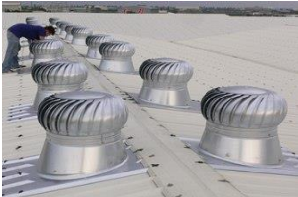
fig App.D.11 (left) | air outlet via roof-openings with rooftop fans (own image) fig App.D.12 (right) | rooftop fans for ventilation (air outlet) (Get Kaung Enterprise Co., 2011)
