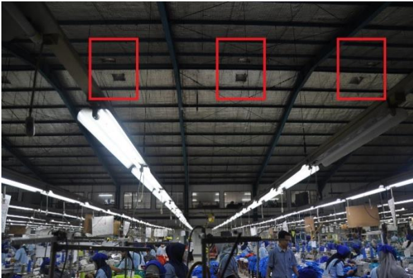
fig App.D.11 (left) | air outlet via roof-openings with rooftop fans (own image) fig App.D.12 (right) | rooftop fans for ventilation (air outlet) (Get Kaung Enterprise Co., 2011)
