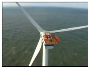
Figure 2.3 Hoisting deck on top of a nacelle
