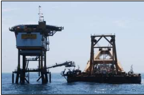
Figure 8.1 Ampelmann at platform decommissioning
