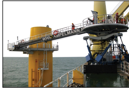
Figure 8.2 Ampelmann at transition piece installation
