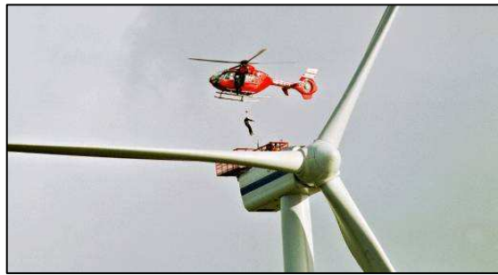
Figure 1.5 Accessing a wind turbine by helicopter
