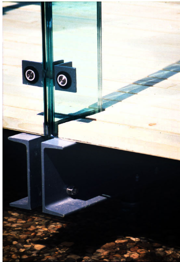
(a) Wall panel - wall panel - glass fin connection in the Glaspavilion (1990), from [23]
