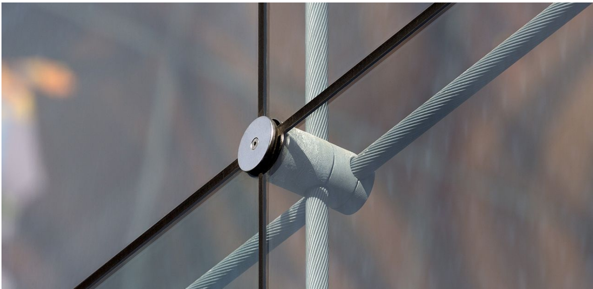
Figure 5.1: Clamp connections in the facade of the Markthal, Rotterdam [28]
