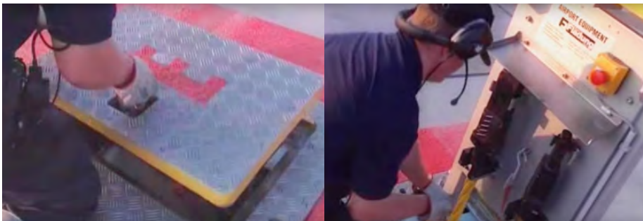
Emirates Engineering's underground technical pits (Haridas, 2012)
