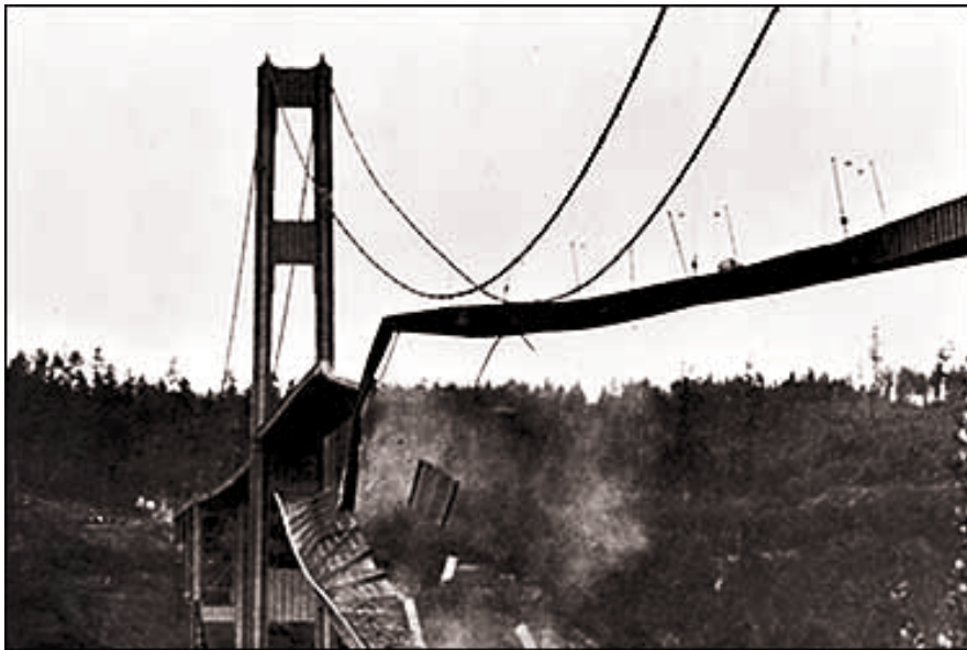
Figure 1-2: Tacoma Narrows Bridge failure due to galloping
