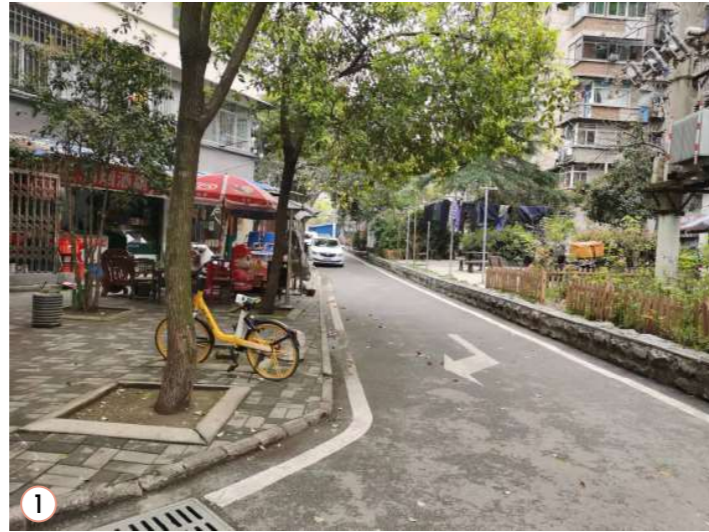
Deteriorated street infrastructure
