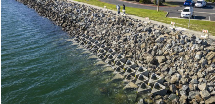
Figure 2. Inaugural deployment of Coastallock unit at the Port of San Diego (PoSD)
