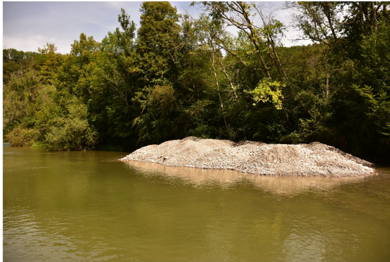
Figure 2. Deposit I in the river before the flood experiment. Its dimensions correspond to ca. 22 \times 8 \times 1.5 \text{ m}^3 (length, width, height). The material was excavated from the adjacent riparian forest. Image © Elena Battisacco.
