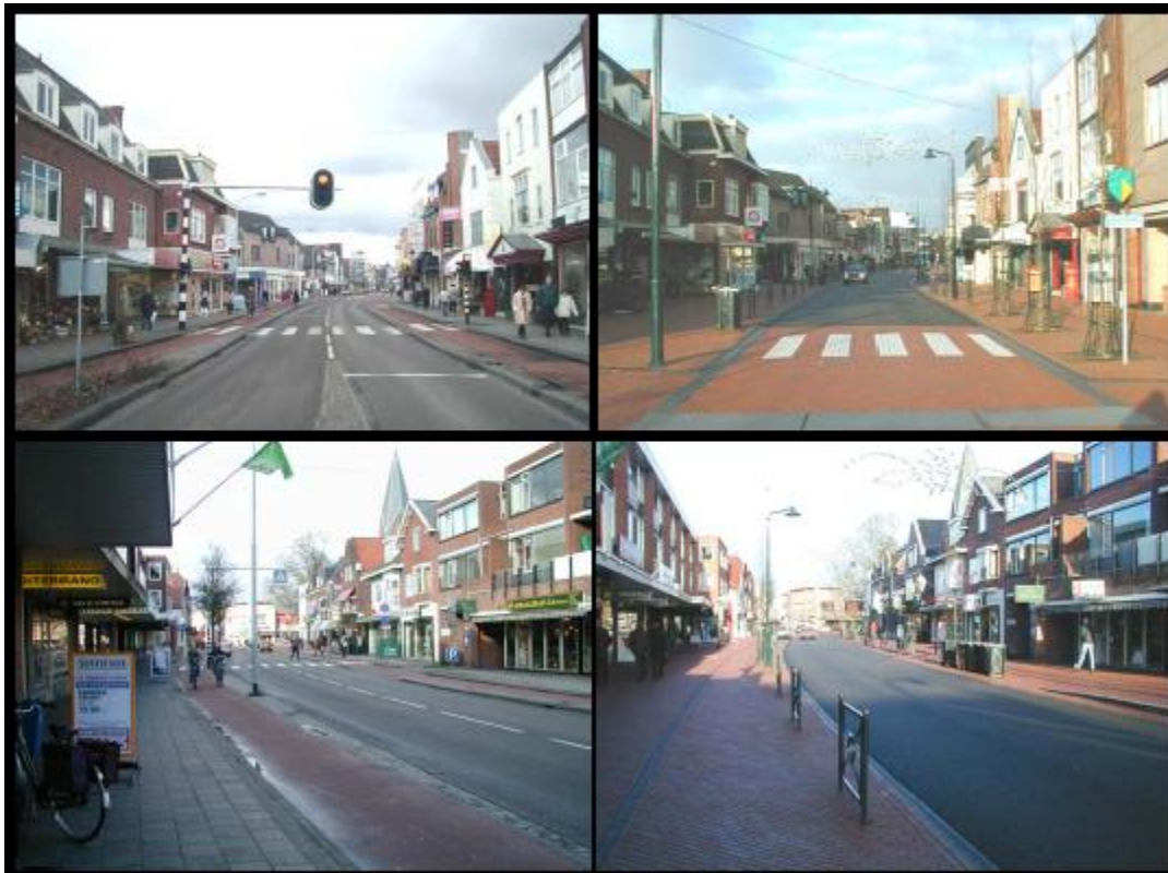
Figure 5.2: Two sections of the road before (above) and after (below) implementing shared space (source: van der Velde and Bos, 2008)
