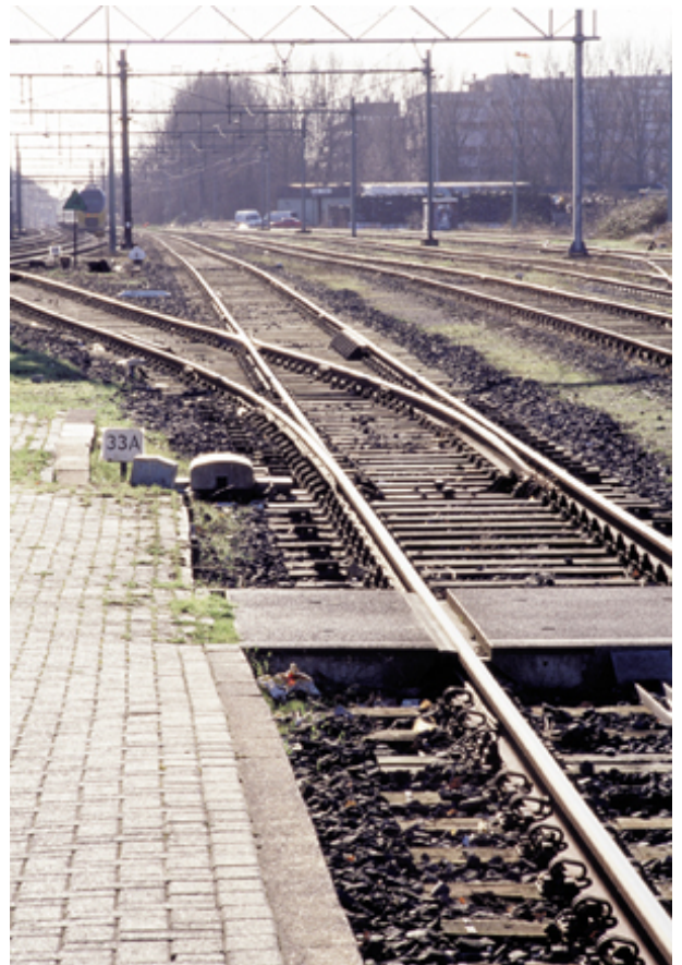
The moveable tongues of a set of points consist of two rails that are fixed in place at one end at what is called the frog and that can slide sideways at the other end. The tongues are not hinged, but bend along their length.
