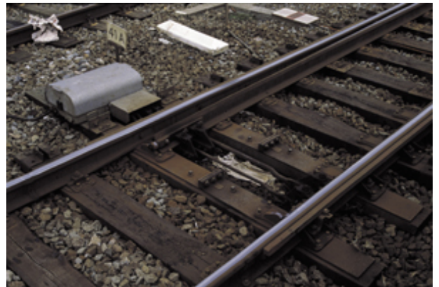
Switching points is done using a points actuator that uses two rods to simultaneously pull the two tongues to one side. The tongues move about 12 centimetres from side to side.
