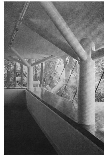
Fig.8 The Grianan building provides glare-free daylight with inwardly sloping glass and upwardly sloping ceilings. Source: U. K. Building Studies
