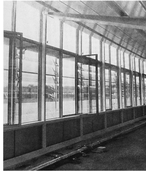
Fig.4 Water-heated framing technologies by Gartner Industries. Source: German Building Studies
