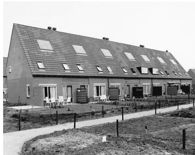
(9) Family homes in Holendrecht-East, Gaasperdam area Source: Stads Archief Amsterdam (unknown) from Gemeente Amsterdam (2018)
