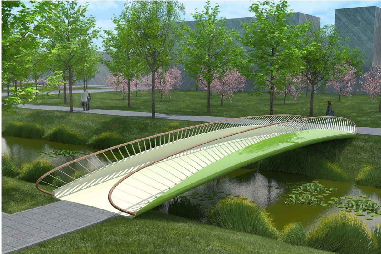
Figure 8: The Delft Design Composite Bridge for pedestrians and bicycles. [Royal HaskoningDHV, FiberCore, 2008]
