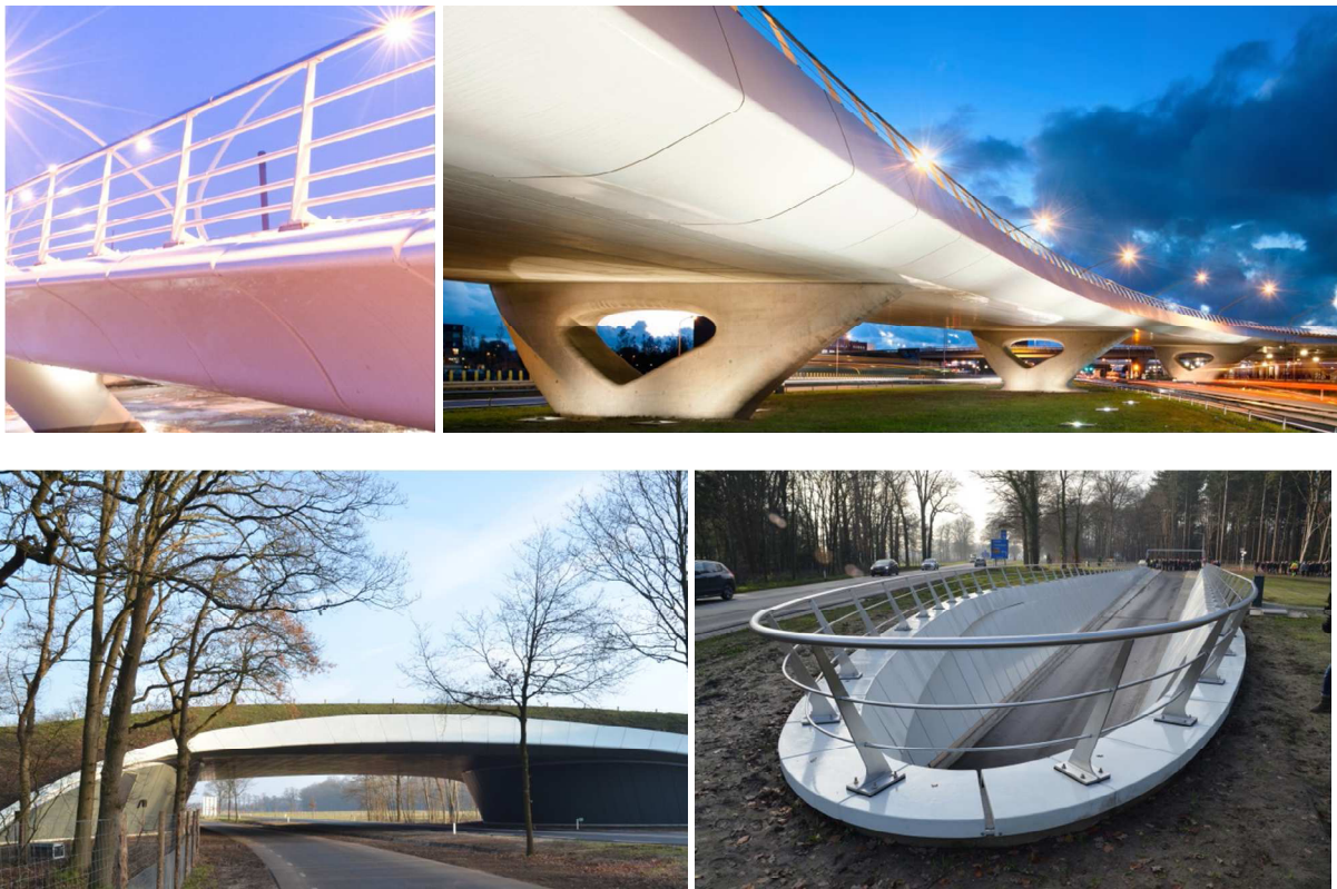
Figure 6: edge elements on the Juliana Bridge in Zaanstad (top left), the fly-over Waarderpolder in Haarlem (top right), and the wildlife crossing and tunnel in Rijssen-Wierden. [Royal HaskoningDHV, 2007, 2013, 2013]
