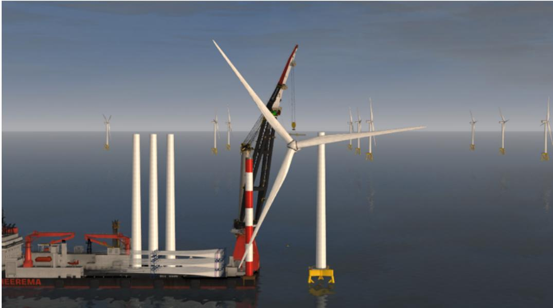
Figure 2.1: Lifting the RNA from the assembly tower to the WTG tower.
