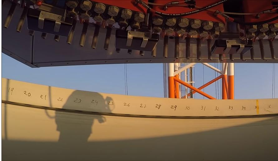
Figure 1.8: Bolt-hole alignment of the nacelle and tower (Fred. Olsen Wind Carrier, 2017).
