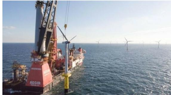
Figure 1.6: Aegir from Heerema Marine Contractors (monohull) installing the DOT offshore wind turbine (HMC).
