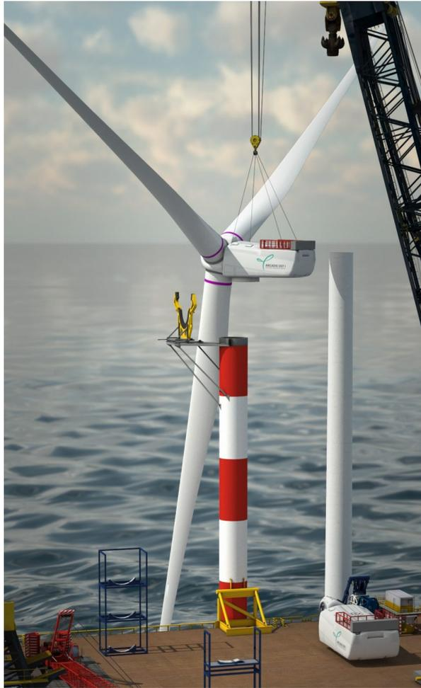
Figure 1.7: Lifting the RNA from the assembly tower on deck of the installation vessel to the already installed tower.
