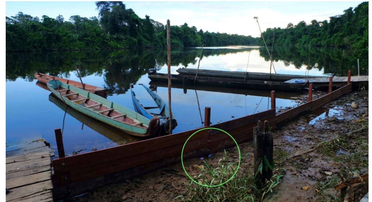
Figure 25: Holes at the bottom of the sheet pile wall
