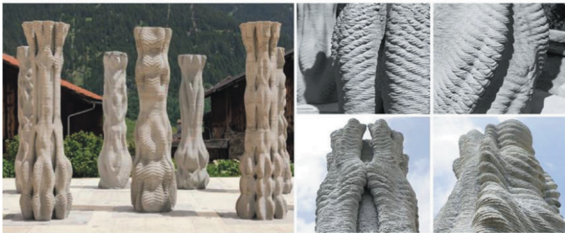
Figure 1. Left: 3DPC columns with column C7 in the middle. Right: 3DPC component details and material tectonics (Anton et al. 2020).
