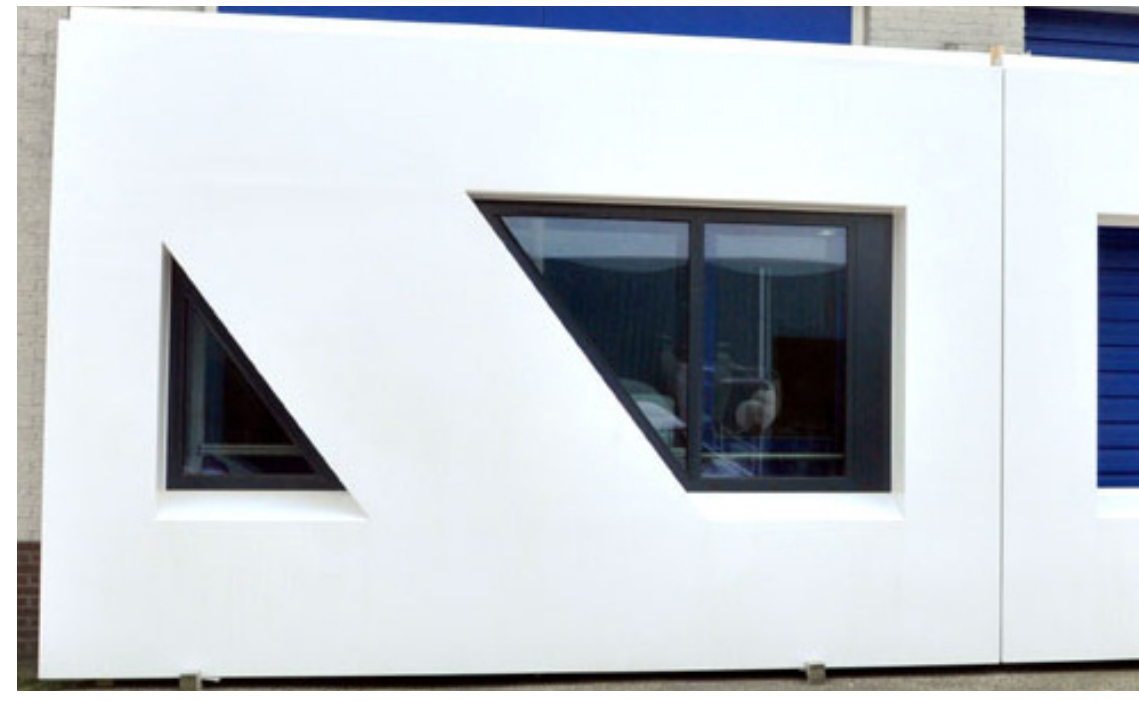
One element of the composite facade
