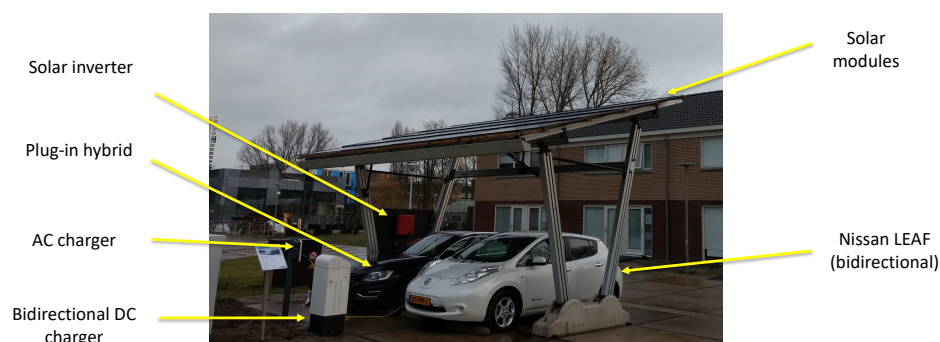
Figure 4: Prototype V2G system at the Green Village (Ghotge, n.d.-b)
