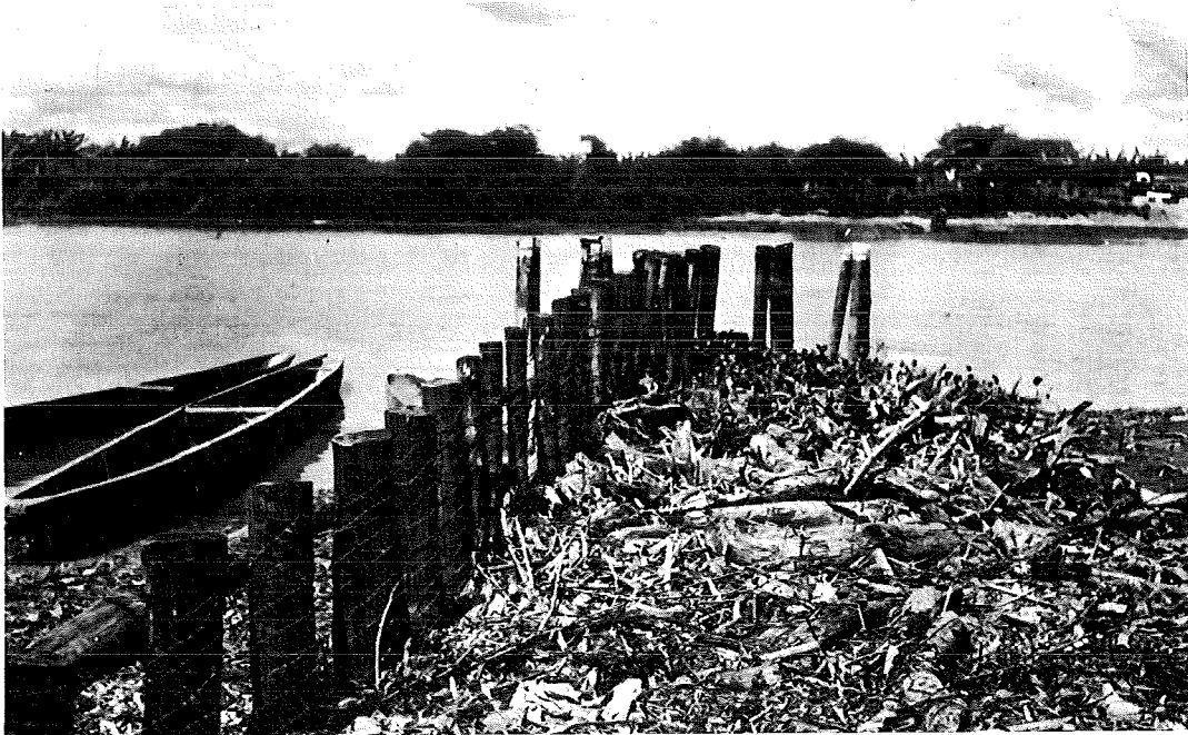
Figure 2.5.12 Open Groyne along the Canal del Dique
